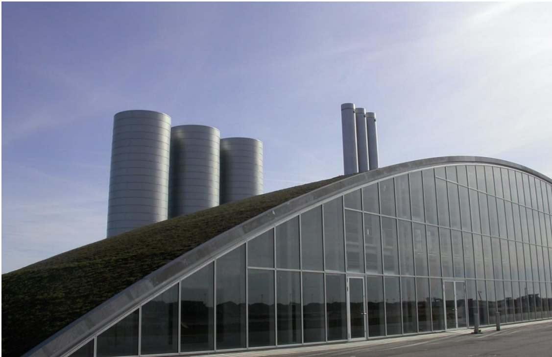
Photo: CTR Peak Load Station by the Copenhagen Airport
